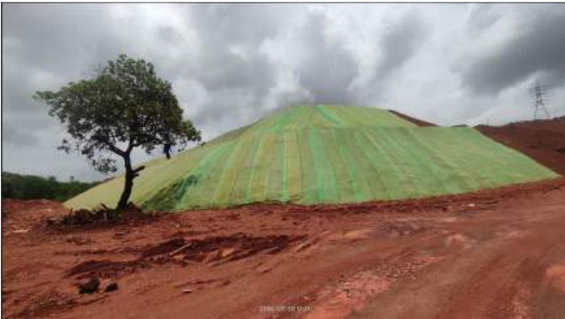
Geotextile Covering
