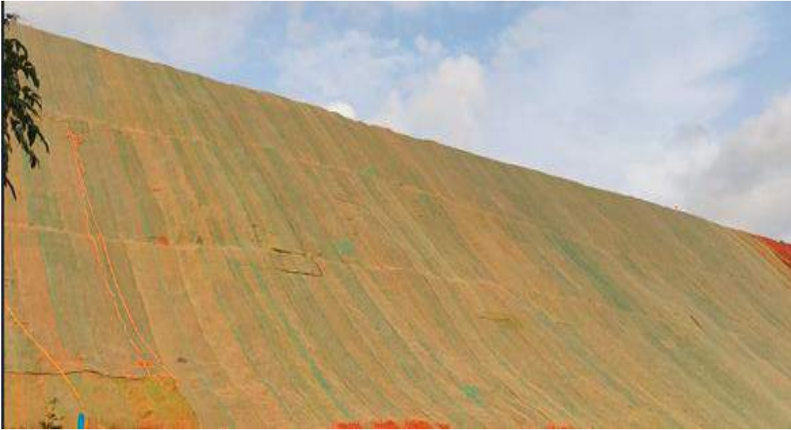
Geotextile Covering
