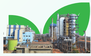
Waste Heat Recovery Power Plant
