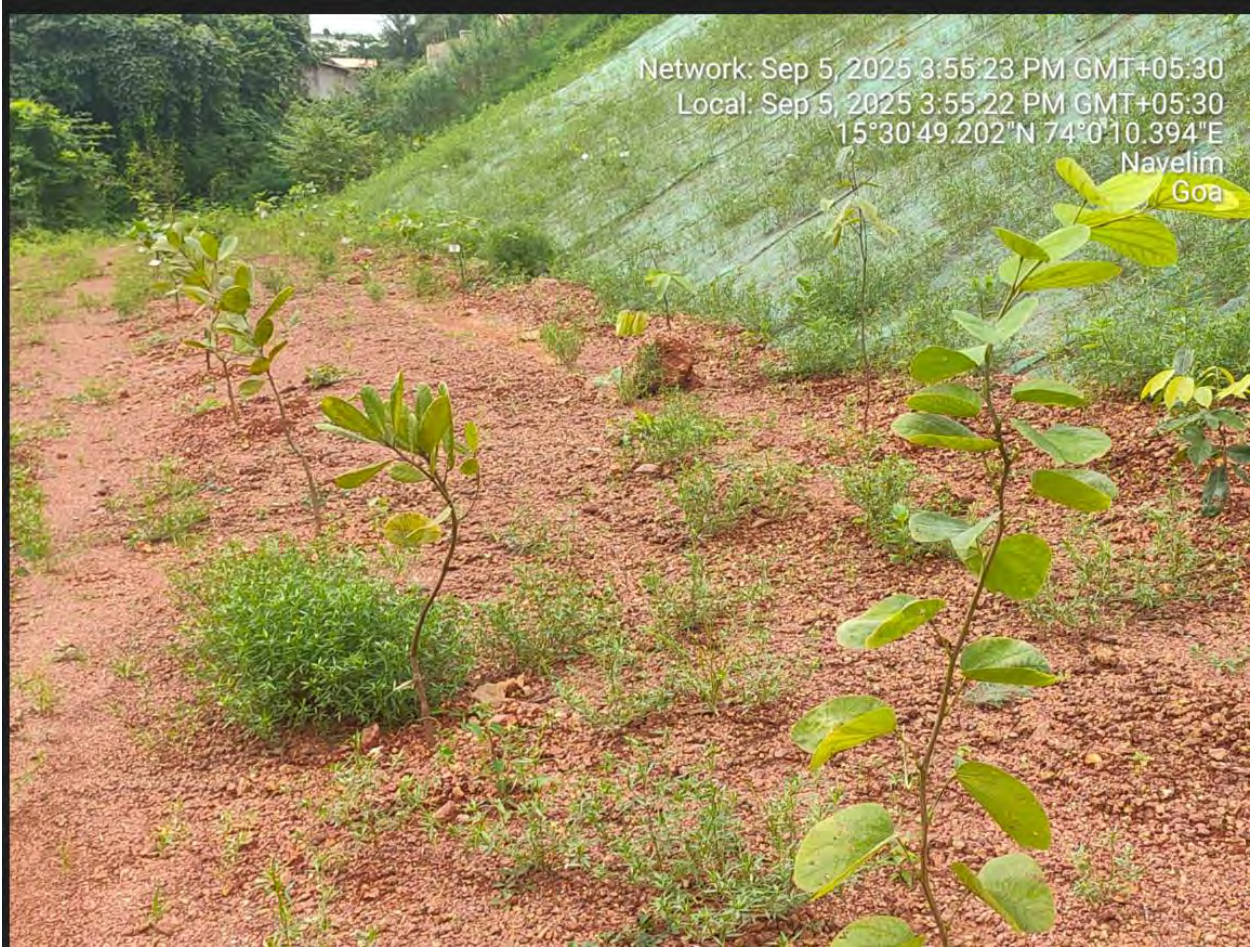
Plantation at the toe of geo textile covered dump
